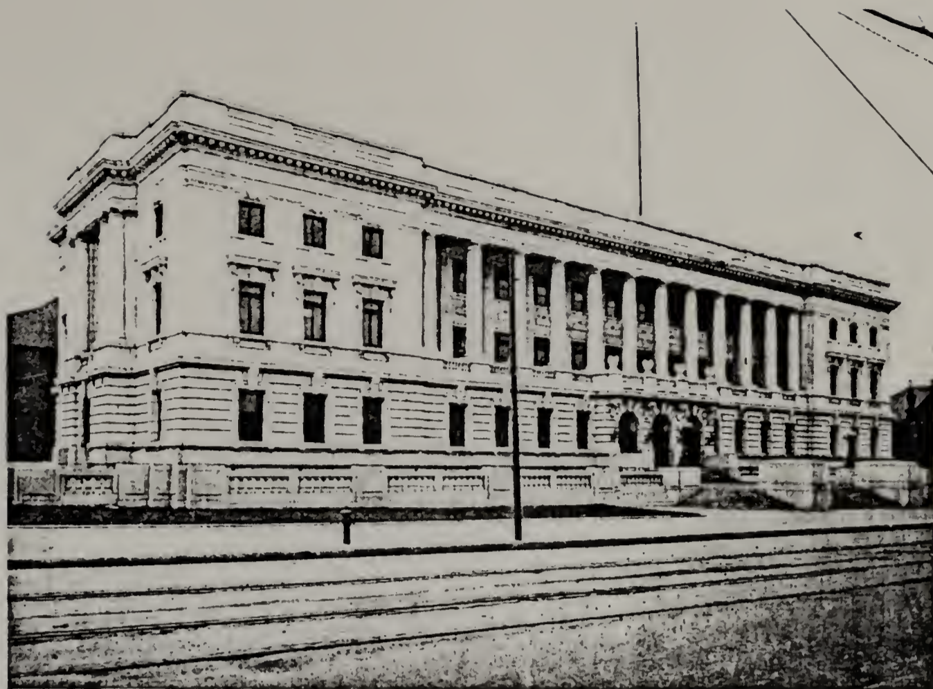
The Present City Hall of Trenton, Completed in 1910, of Which Ferdinand W. Roebling Was Chairman of the Building Commission
